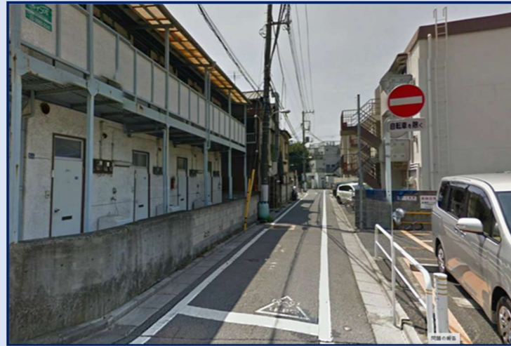
●道路拡幅整備前 ②
