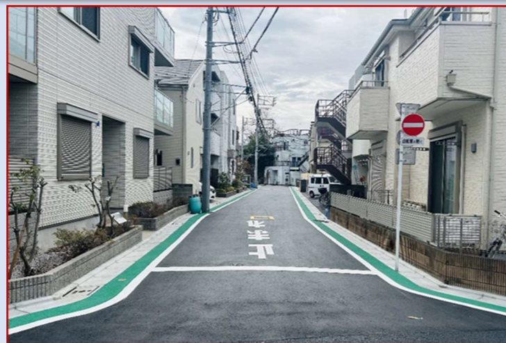
●道路拡幅整備後 ②
