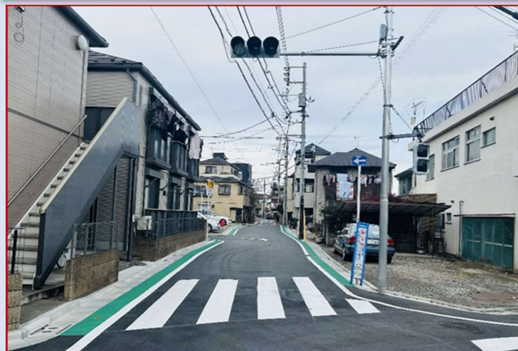
●道路拡幅整備後 ①
