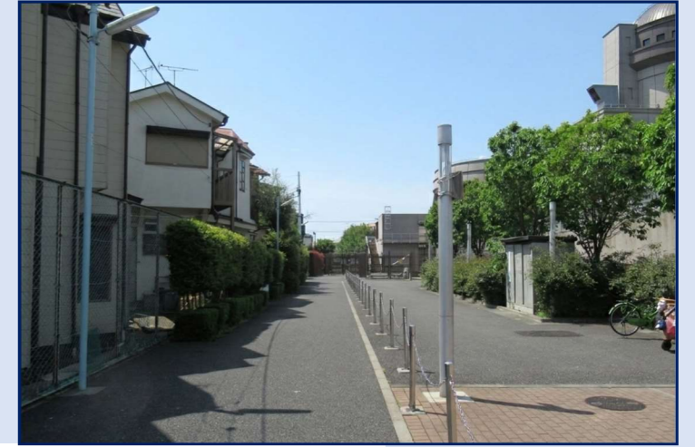
●道路拡幅整備前 ④
