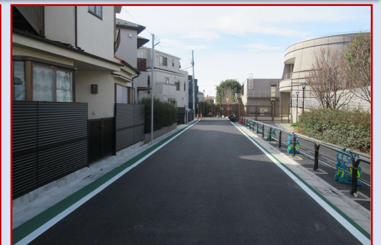
●道路拡幅整備後 ④
