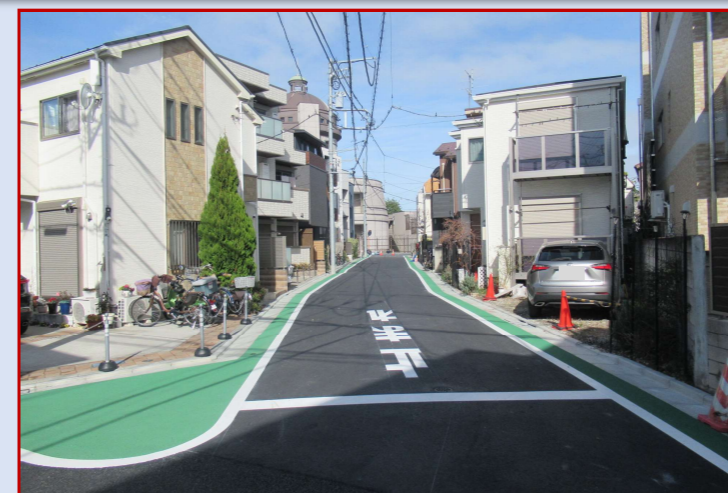
●道路拡幅整備後 ③
